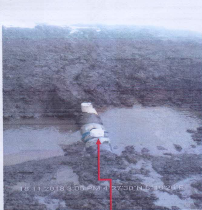
Fig C: Incident Facility after repair
